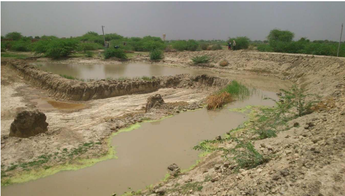
Near to Completion
