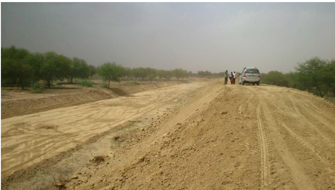
Near to Completion
