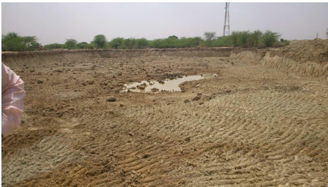
Near to Completion
